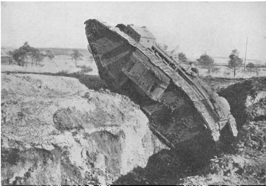
Fig. 235.—Tank Climbing with Assistance of Unditching Gear
