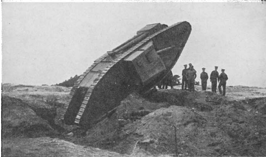
Fig. 234.—Tank at about Maximum Climbing Angle
